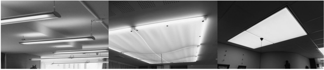
FIGURE 21.2 (See color insert.) Examples of dynamic lighting installed in Dutch nursing homes: Amadea by Derungs (left), Biosun by Van Doorn (middle), and Strato by Philips (right).
