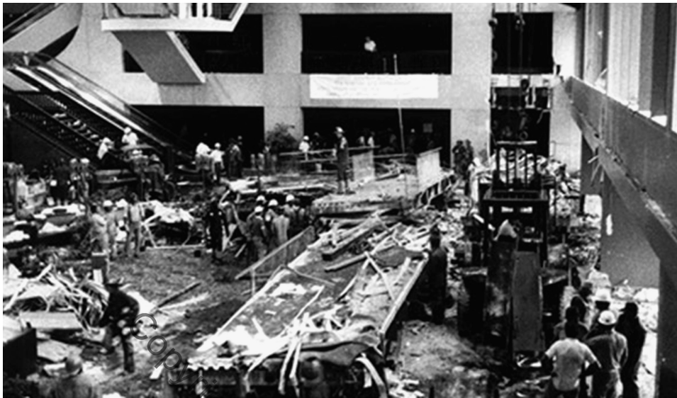
Figure 1.1 Wreckage of the collapsed Hyatt Regency Hotel in Kansas City. (Associated Press file photo. With permission.)
