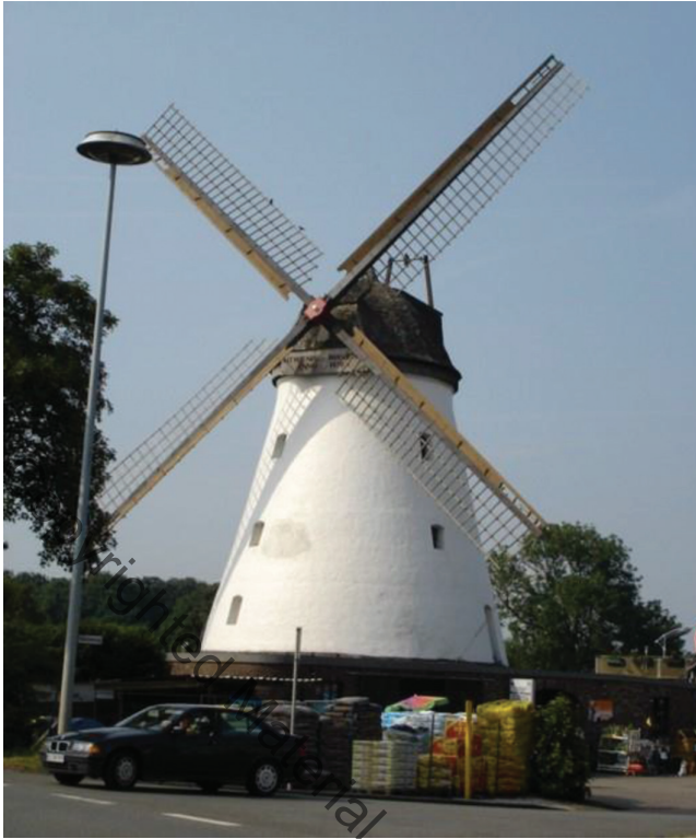
FIGURE 1.1 Renovated nineteenth-century windmill.
