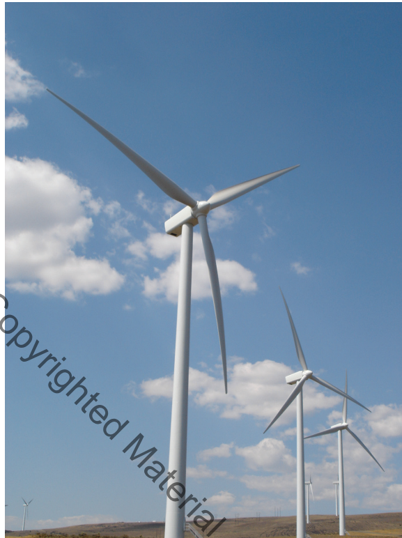
FIGURE 1.7 A 1.8 MW horizontal-axis wind turbine.
