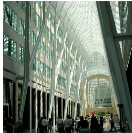
Figure 40: Allen Lambert Galleria , Toronto: a structure that provides natural light but necessitates shading to counteract direct solar heat gain
