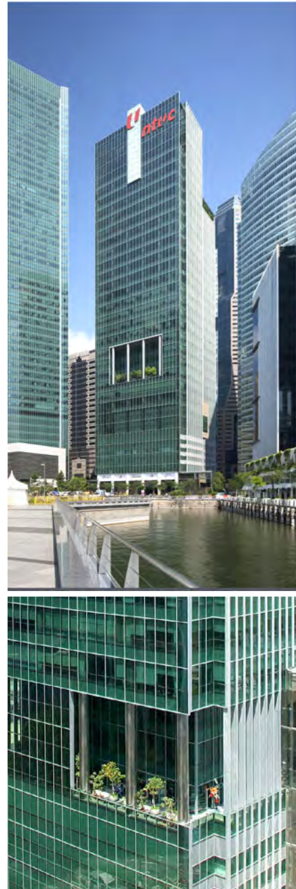
Figure 59 (top-bottom): NTUC, Singapore: an example of how at least 60% of the area of the skycourt should be kept open with low walls
