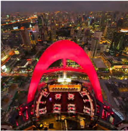
Figure 54: Red Sky , Bangkok: A rooftop restaurant that manipulates views of the Bangkok skyline to be an income-generating destination
