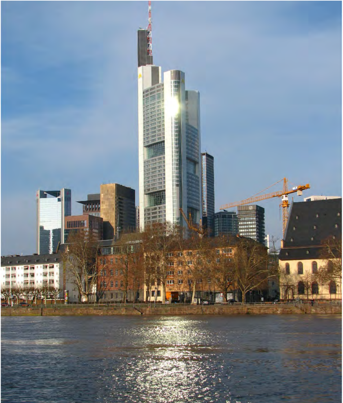
Figure 26. Commerzbank , Frankfurt an exemplary environmentally responsive building that incorporates skycourts to form a vertical working village
