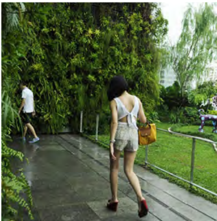
Figure 42: Orchard Central, Singapore: applying vertical greenery to reduce heat and noise generated by mechanical plant areas
