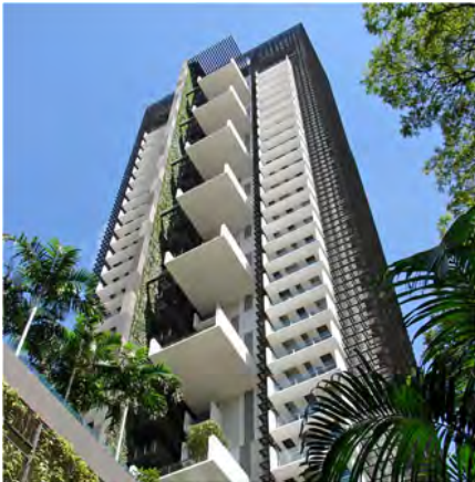
Figure 58: Newton Suites , Singapore: an example of skycourts acting as communal space that would be exempt from overall development area calculation
