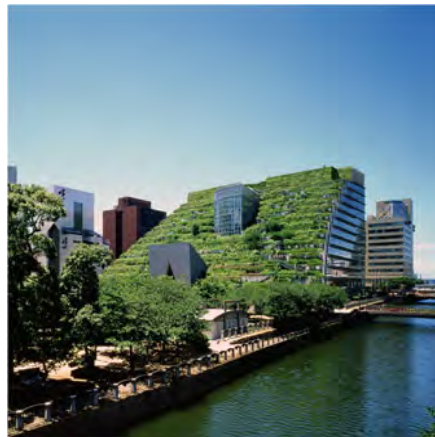
Figure 41: Acros Building , Fukuoka: greening vertical and horizontal surfaces can help reduce ambient temperatures
