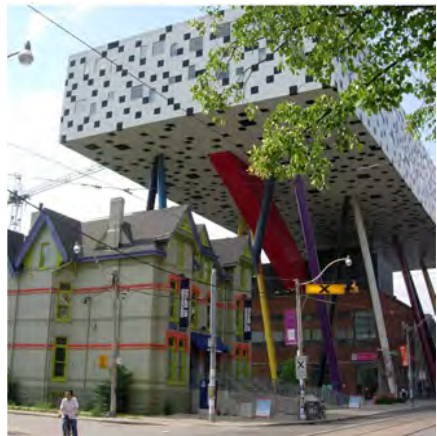
Figure 53: Ontario College of Art and Design, Toronto: exploiting the air rights above an existing building to increase density
