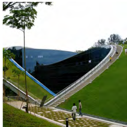
Figure 52: Nanyang Technical University, Singapore: the green roof as a means of reducing energy consumption
