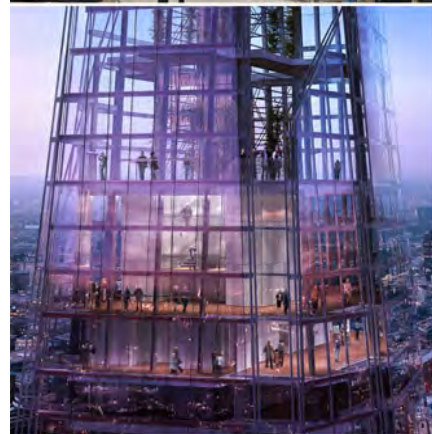
Figure 39: (top–bottom) The Shard , London: its mid-level skycourt acts as a transitional space as well as a destination space
