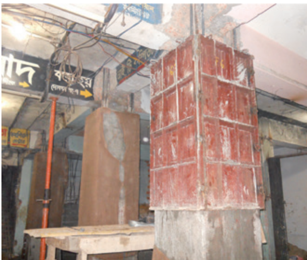
Structural re-enforcements in an Accord factory building
