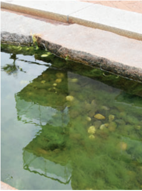
Storm water catchment strategies have been designed into the public realm throughout the Western Harbour District
